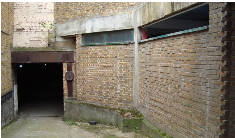
Figure 3 - Access to a car park beneath London Wharf
