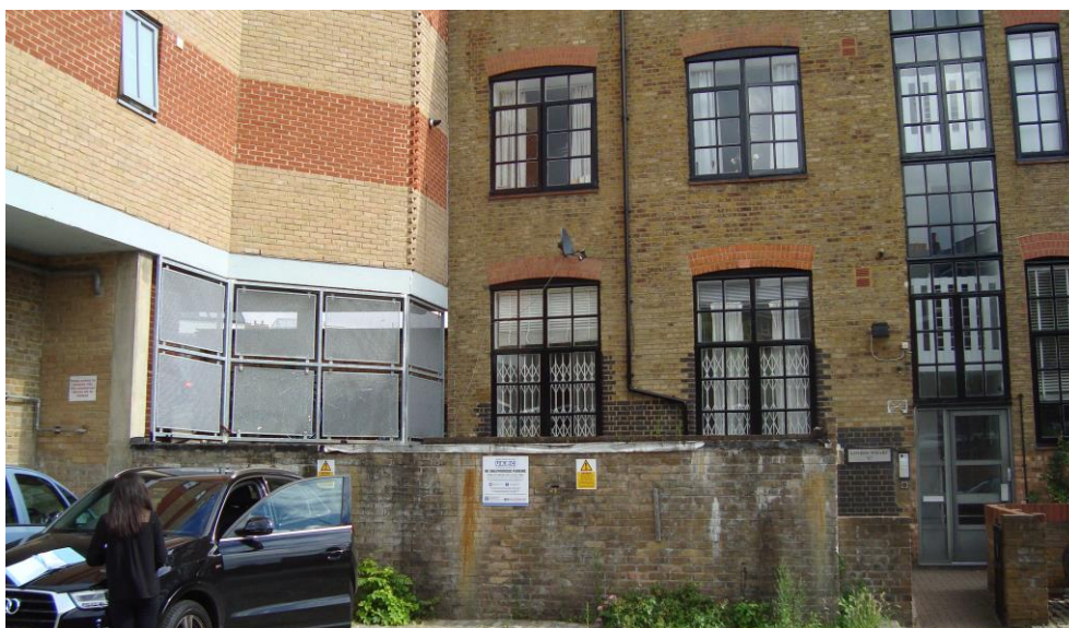
Figure 4 - single storey brick built structure in front of London Wharf to be demolished
